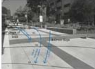
Diagram of a sloping walkway at Grand Park in LA. The walk has a primary 4 percent slope and was designed with a cross slope to ease surface water to the planting area.
