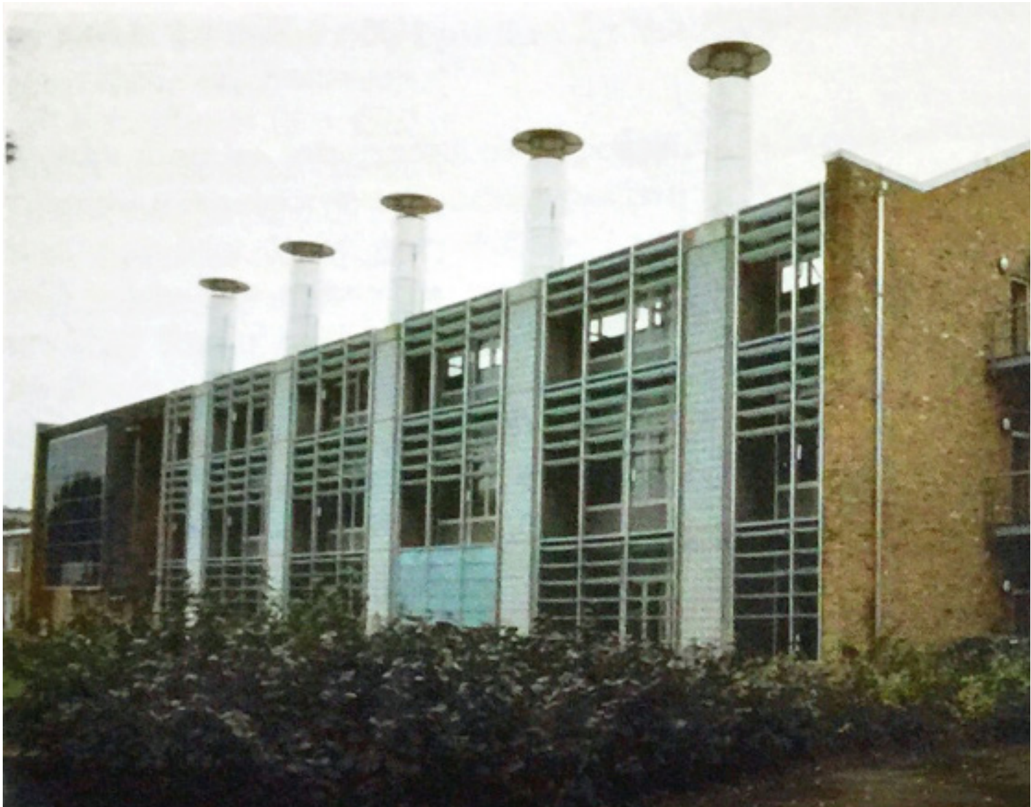
02 Solar chimneys at the Building Research Establishment office, Garston, Hertfordshire, UK. THERESE PEFFER
