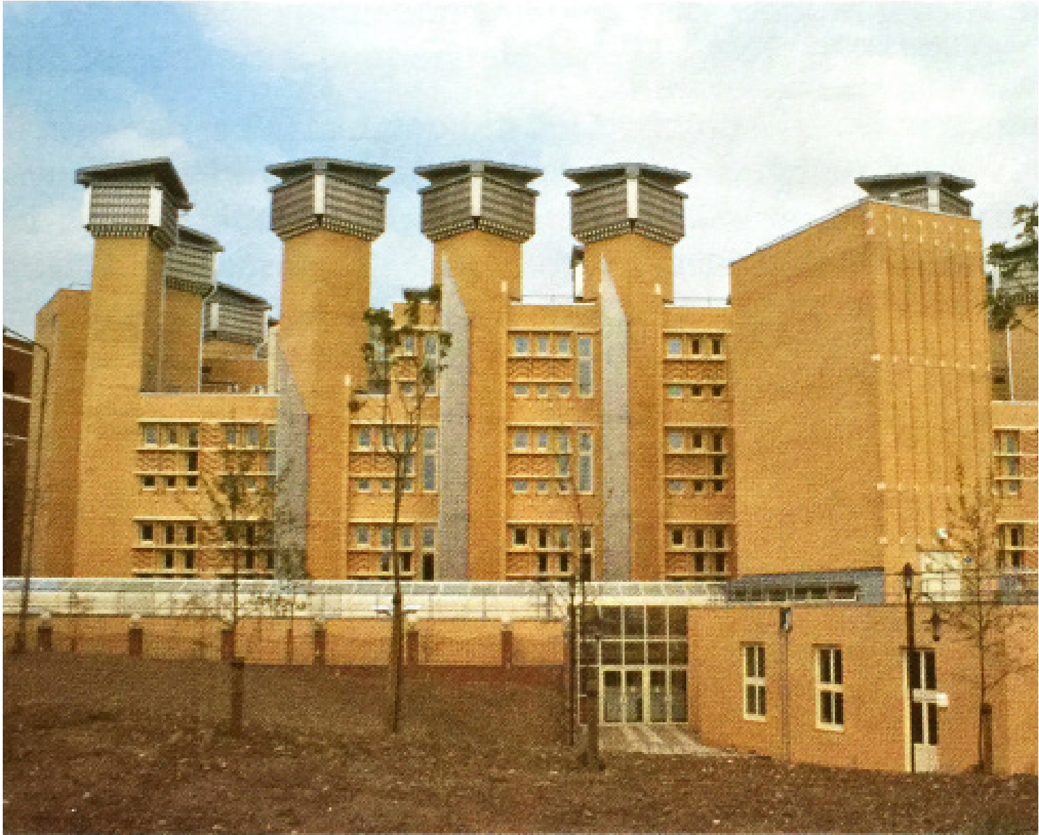
The Eastgate Centre in Harare – A Termite Mound In Disguise (Left) Termites use dense materials that store heat in the day. They then use specific methods of ventilation to remove heat at night. Architect Mick Pearce studied the termites’ movement and use of space, mapping the structure of their tunnels and galleries . Stack ventilation towers exhaust warm air at Lanchester Library at Coventry University, Coventry, UK. (Above) Stacking effect providing more air movement (ventilation) at lower levels of a stack, while modular and separated stacks can address this problem. But on the other hand, we also need to consider about cost, opening requirement, etc.
