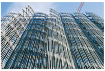
WEST FACADE- REEDS COVER THE FACADE
