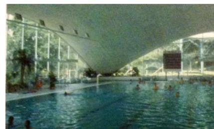
Shells spring from the foundation and continuously curve over to envelop interior space.
