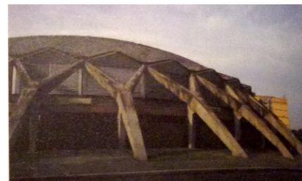
Shells does not meet the foundations directly but ends at the eaves level where inclined struts resist the outward thrusts
