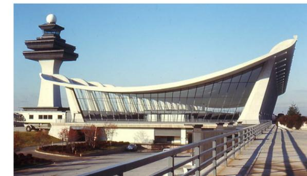
Catenary structures transfer loads to their supports through tension, which are usually made by concrete struts or steel masts.
