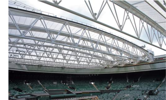
Trusses are prefabricated and placed on struts which transfer the load to the foundation. Struts of this structure can be concrete, wood or steel.
