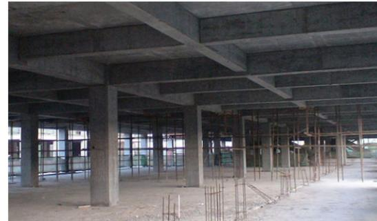
Framed structure consists of beams and columns. Columns play an important role bearing load in framed structure.
